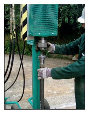
28. To add additional rods use the Rod Spanner to suspend the drill string in the borehole.
