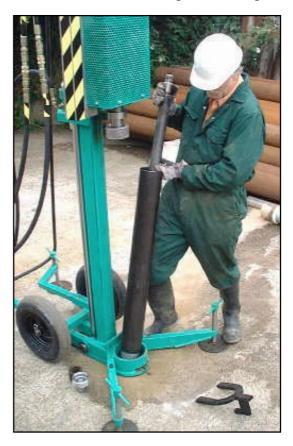
38. Attach the casing drive head, and drive ring (the spacer tube is not required after the first metre). Connect to the rig using the bottom adaptor.
