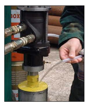
17. Start rotating the core bit by engaging the Right-hand lever on the control block.
