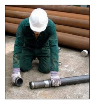
36. Drop the empty sampler down the hole and remove the casing drive head.
