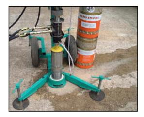
19. Ensure that water is flushing the bit continuously during coring. If water circulation stops, remove the core bit from the hole to prevent it becoming burnt out.
