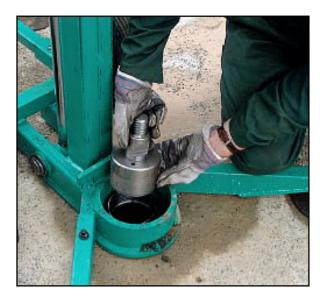
42. Withdraw the casing from the ground and secure with casing slips before uncoupling.
