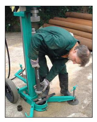
41. To remove the casing from borehole, remove the casing drive head and attach the lifting head.
